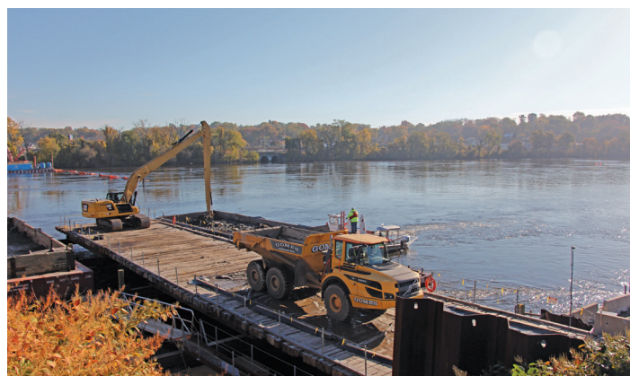
RIVER CROSSING Crews hauled dredged material across the river by barge for removal and temporary storage on site.
