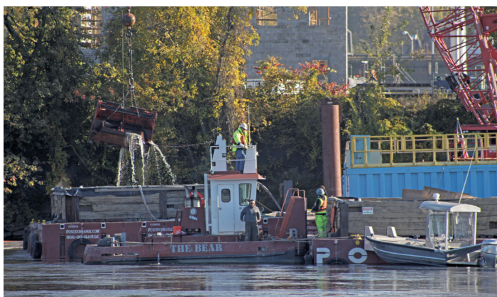
DREDGE REPORT The project's dredging operation began excavating the 59-ft-wide by 15-ft-deep trench from the east side of the river working toward the west for the pipelines from the pump station to the treatment facility in December 2021.
